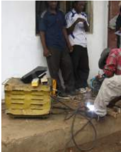
Figure 5 Existing welding machine being tested on site in Kilosa
